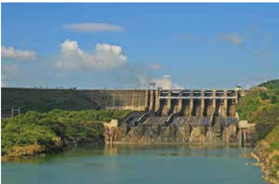
The 360MW Magat HEPP of SN Aboitiz Power – Magat, Inc., a joint venture between Aboitiz Power Corporation and SN Power Invest AS of Norway. [Photo courtesy of Aboitiz Power Corporation]
